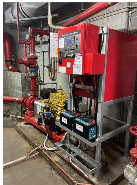
Figure 10: Diesel Sprinkler pump
