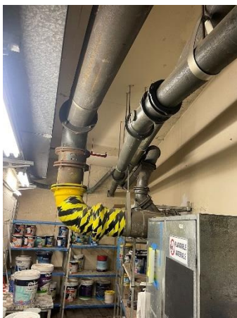
Existing Mild Steel sewer drainage.
