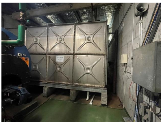
Figure 5: Roof top combined potable/fire hydrant tank.
