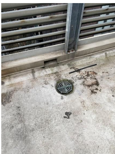
Existing L11 roof stormwater outlet and overflow.
