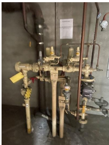
Existing High pressure gas boundary regulator.
