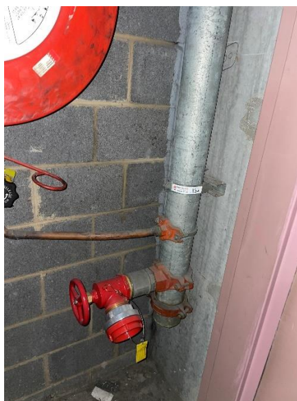
Figure 4: Fire hydrant in cupboard.
