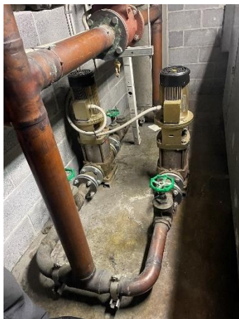
Existing CW. transfer pumps.
