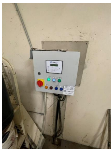
Existing Stormwater pumpstation control panel.
