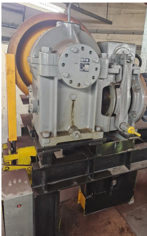
Original as-installed Otis Elevator Geared Machine
