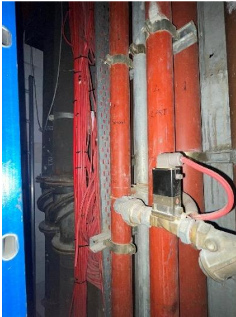
Figure 6: On-floor sprinkler control valve assembly
