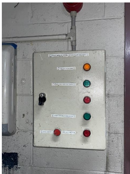
Grease Arrestor level alarm.
