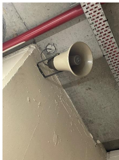
Figure 19: EWIS horn speakers and strobe lights
