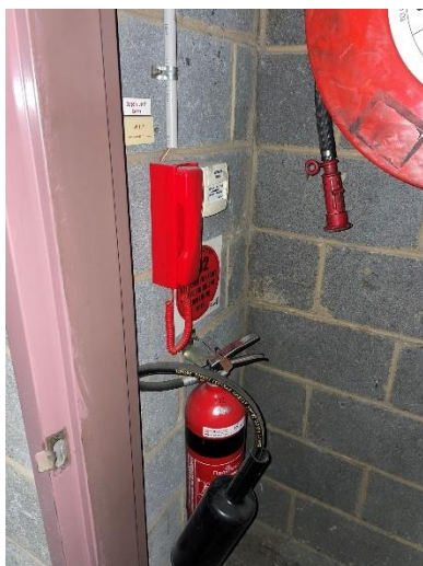
Figure 18: WIP/ECP points within cupboard.
