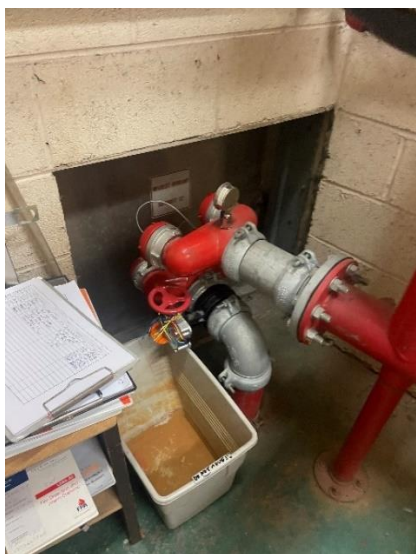
Figure 1: Existing fire hydrant booster assembly
