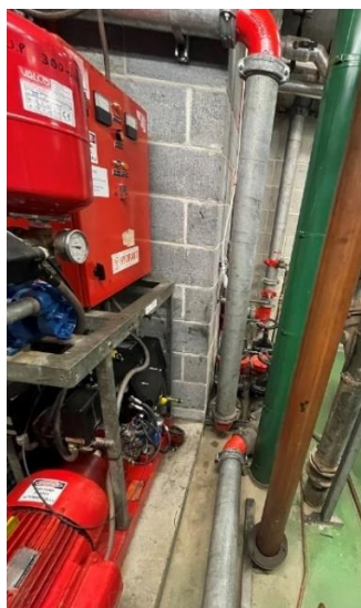
Figure 2: Existing Diesel/Electric Hydrant pump
