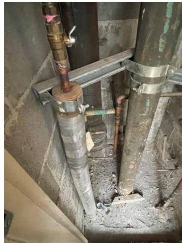
Existing Hot Water services pipework.
