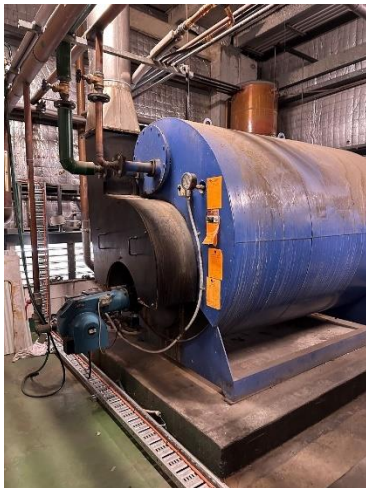
Existing Domestoc HW boiler.
