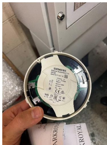
Figure 17: Existing smoke detector.
