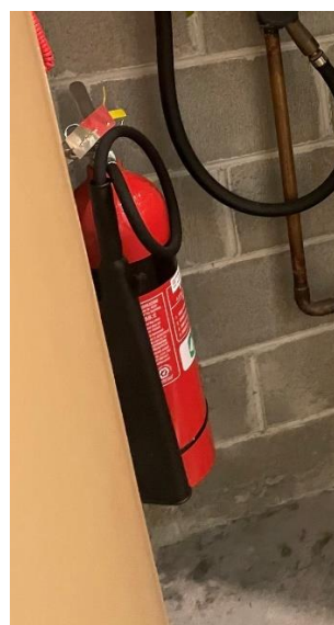
Figure 12: CO2 Fire extinguisher
