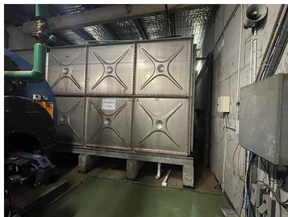
Existing Combined CW. & FH water storage tank.
