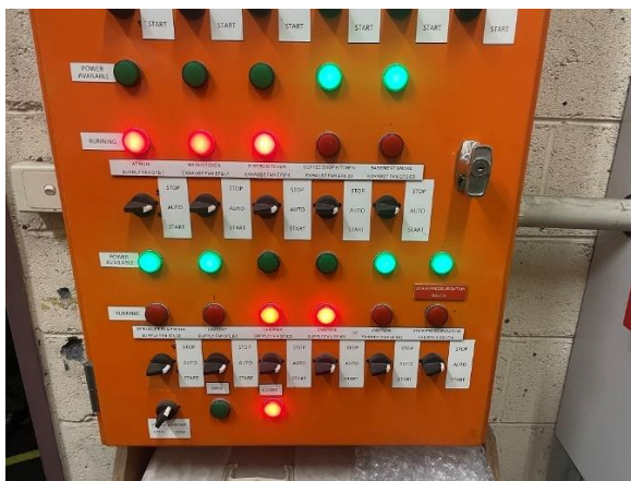
Figure 15: Existing Fire Fan Control panel (FFCP).
