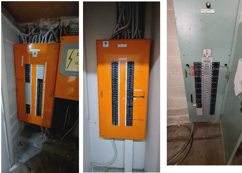
Figure 4-4: Typical Distribution Boards
