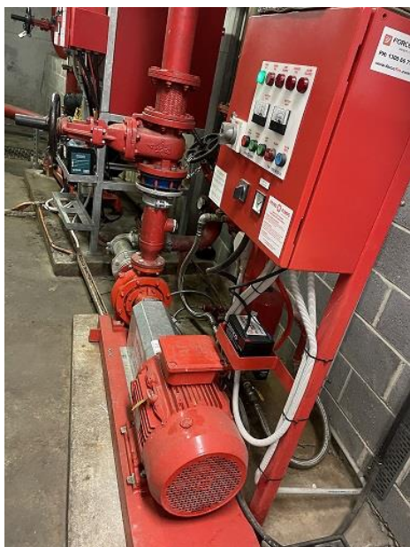
Figure 9: Electric Sprinkler pump
